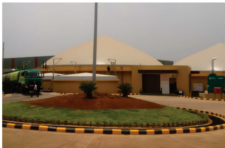
Noble Exchange's state-of-the-art biogas manufacturing plant at Pune
